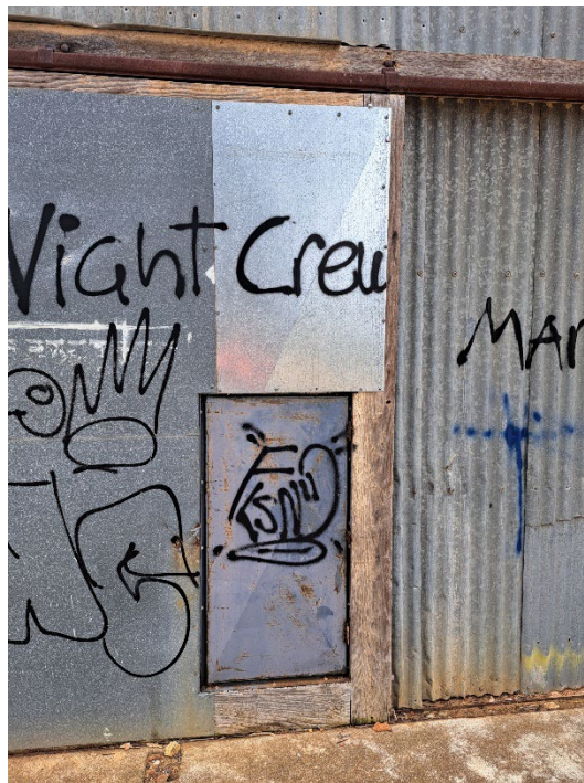
Figure 2: In an attempt to reduce vandalism and unauthorised access Council have welded the pump shed doors shut
