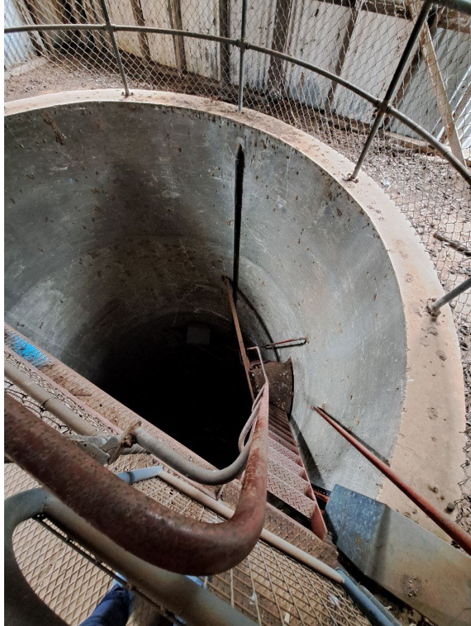
Figure 4: The concrete dry-well structure appears sound, however, the access is not compliant with current safety requirements
