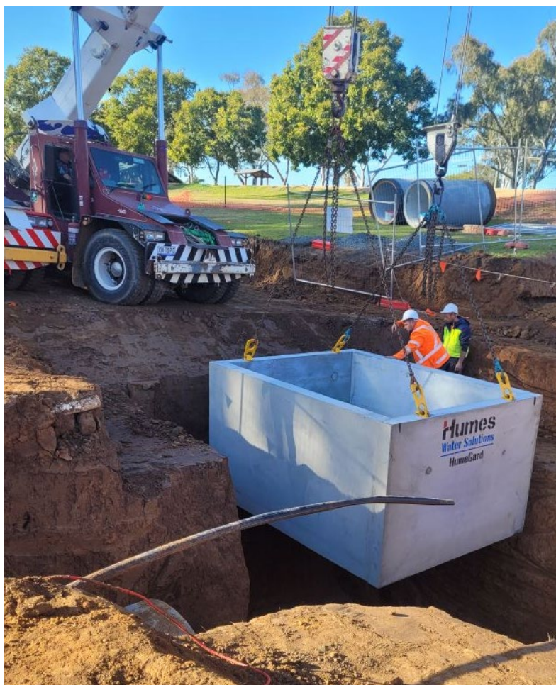
Figure 7: One of the final stages of the pipework installation - the gross pollutant trap was installed at Rotary Park
