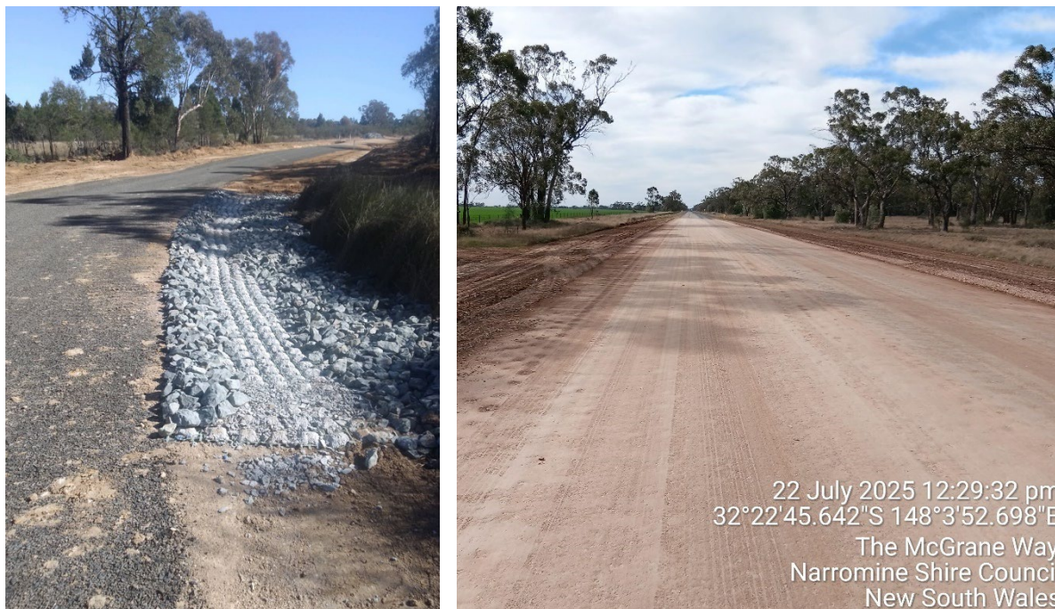
Figure 3: Momo Road improvements - (Left) Council is utilising concrete matting to improve drainage, (Right) Great progress on Tullamore Rd upgrade with next section ready for sealing in August
