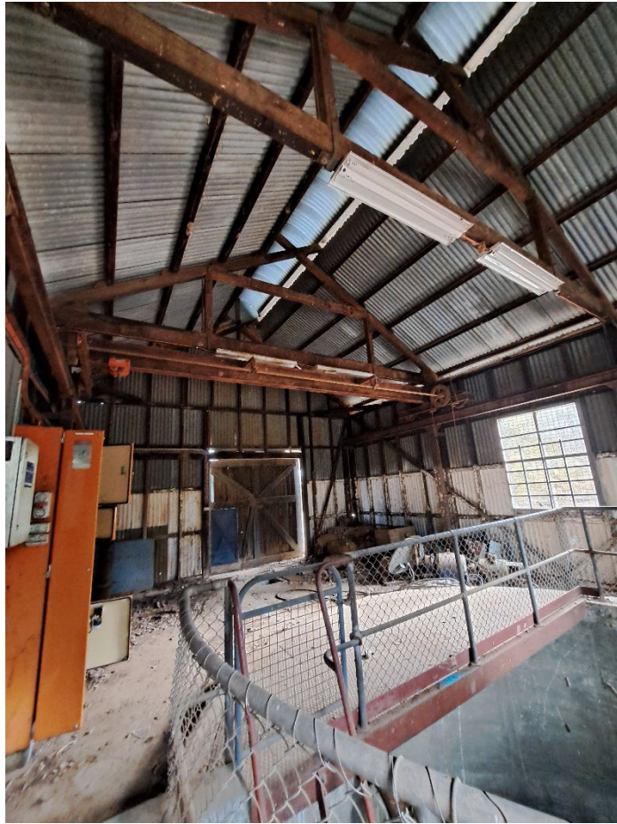
Figure 3: The existing gantry is non-compliant and will require replacement
