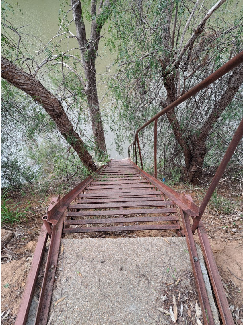
Figure 6: Access stairs to the inlet foot valve are very unsafe, not properly anchored and need replacing
