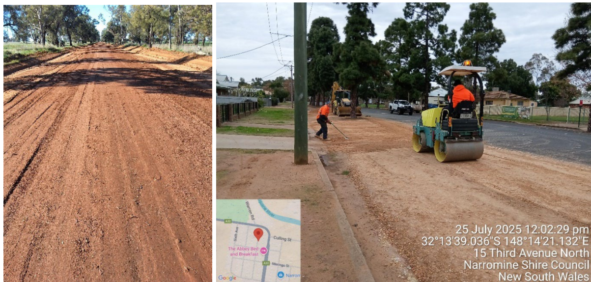
Figure 2: Hamilton's Lane - (Left, )Shoulder/Verge repairs on Third Ave, Narromine -(Right)
