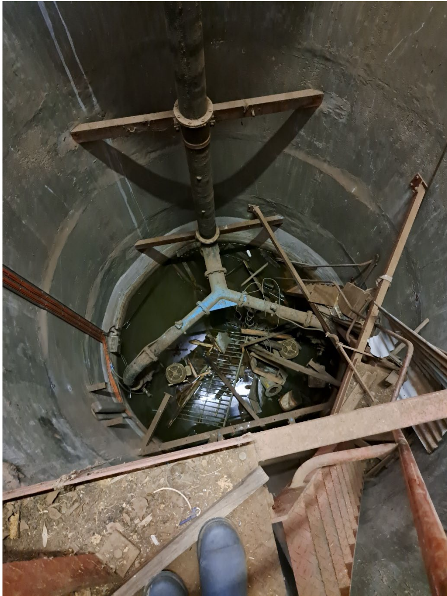
Figure 5: The dry-well has a lot of material from vandalism that requires removal
